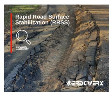
Heavy vehicles are known to cause damage accumulation when traversing weak or damaged pavements. Expedient construction techniques are needed to rapidly improvement structural capacity of roads to support these loads. (Photo courtesy of the ERDC)
